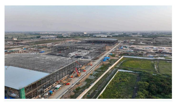
Structural steel framework now nearing completion for Agratas' Sanand battery facility. Tata Group
