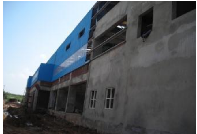
Side Cladding Work Completed
