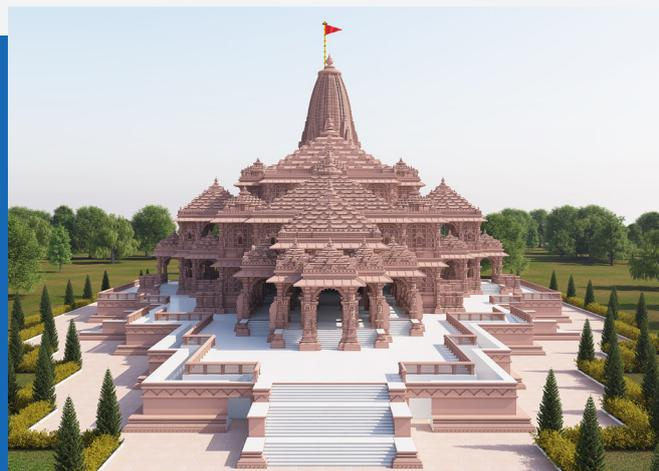
The temple structure will be constructed using a traditional stone structure made up of sandstone. The structural elements are joined together by tongue and groove joints. Its dimensions are approx. 380x250 feet. The main dome over Garbhagriha is 161 feet high.
